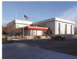
Paso Robles Tank, Inc., Nevada
