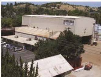
Paso Robles Tank, Inc. Corporate Office
