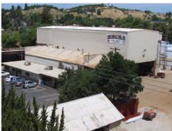
Paso Robles Tank, Inc. Corporate Office
